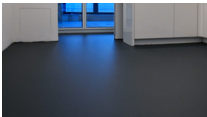
Smooth floor coating in all rooms
