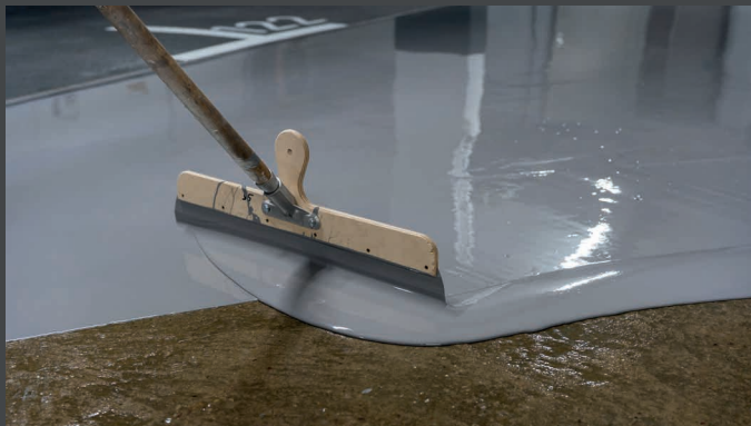
Application of VIASOL PU-L2000
