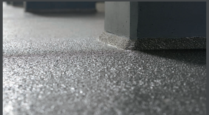
Support pillar floor connection
