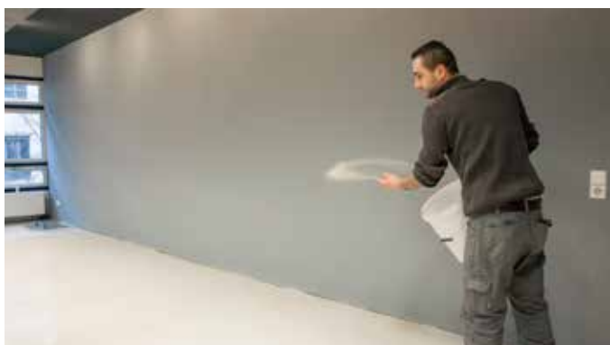
Sanding after applying primer
