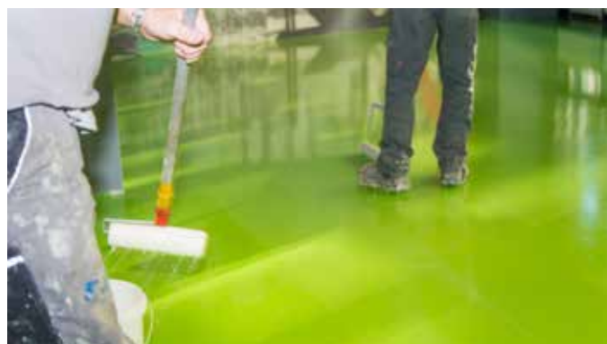
Sealing of the new floor
