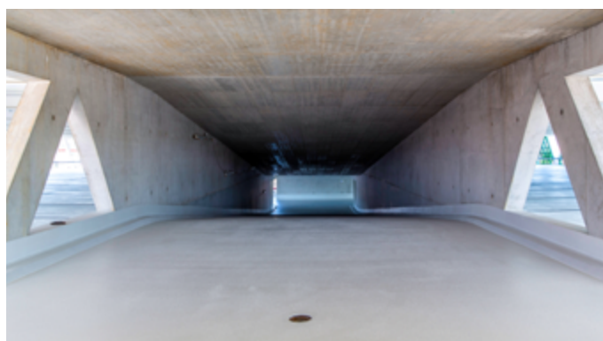
The floor on the ramps was coated with an OS 10
