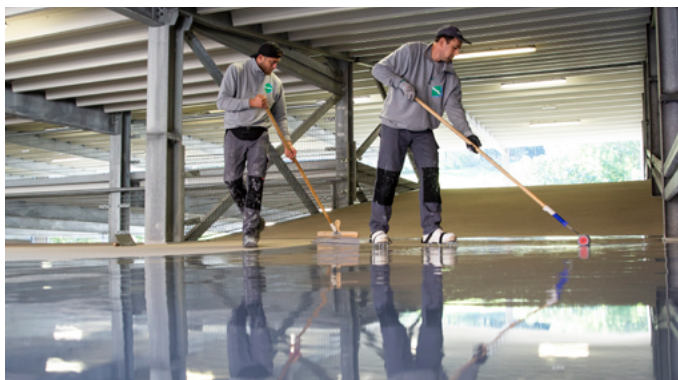
Manual application of the sealing membrane
