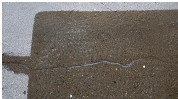
Preparation work sealing the cracks
