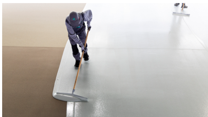
Coating an intermediate level
